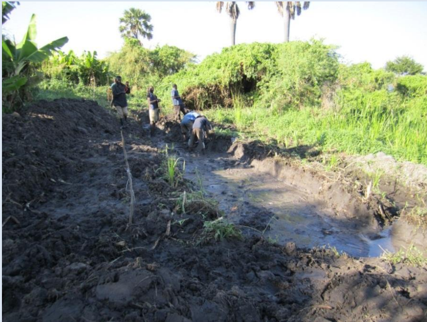
Initial digging of the fish pond
